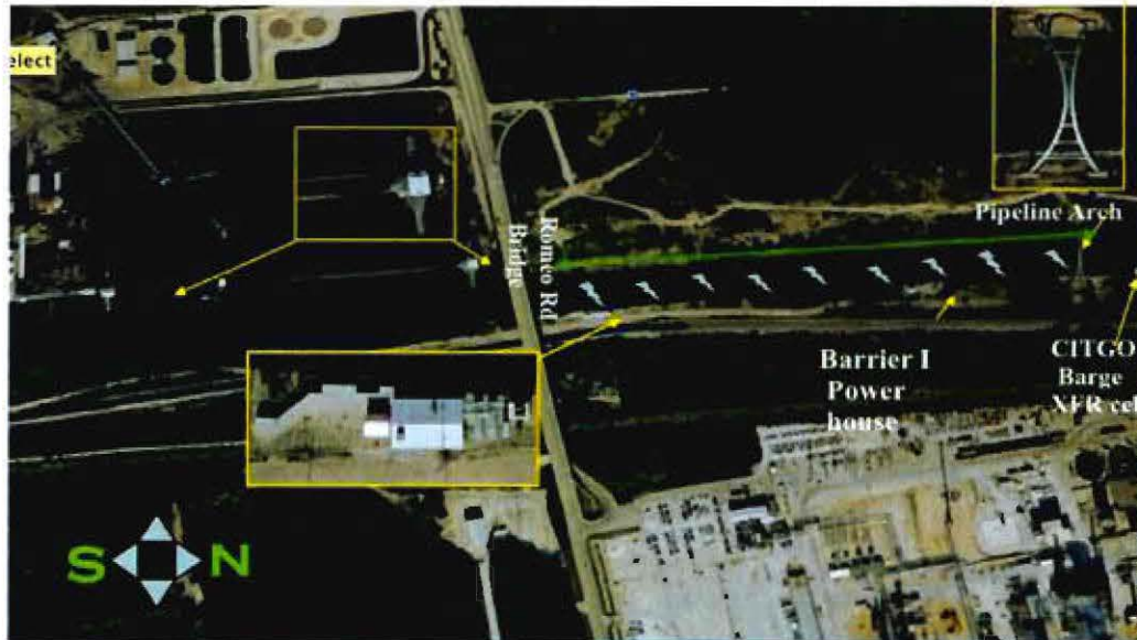
Figure 1: Aerial view of the Chicago Sanitary and Ship Canal Aquatic Nuisance Species Dispersal Barrier (“Barrier I”), located in Romeoville, IL (Source: U. S. Army Corps of Engineers, Chicago District)
